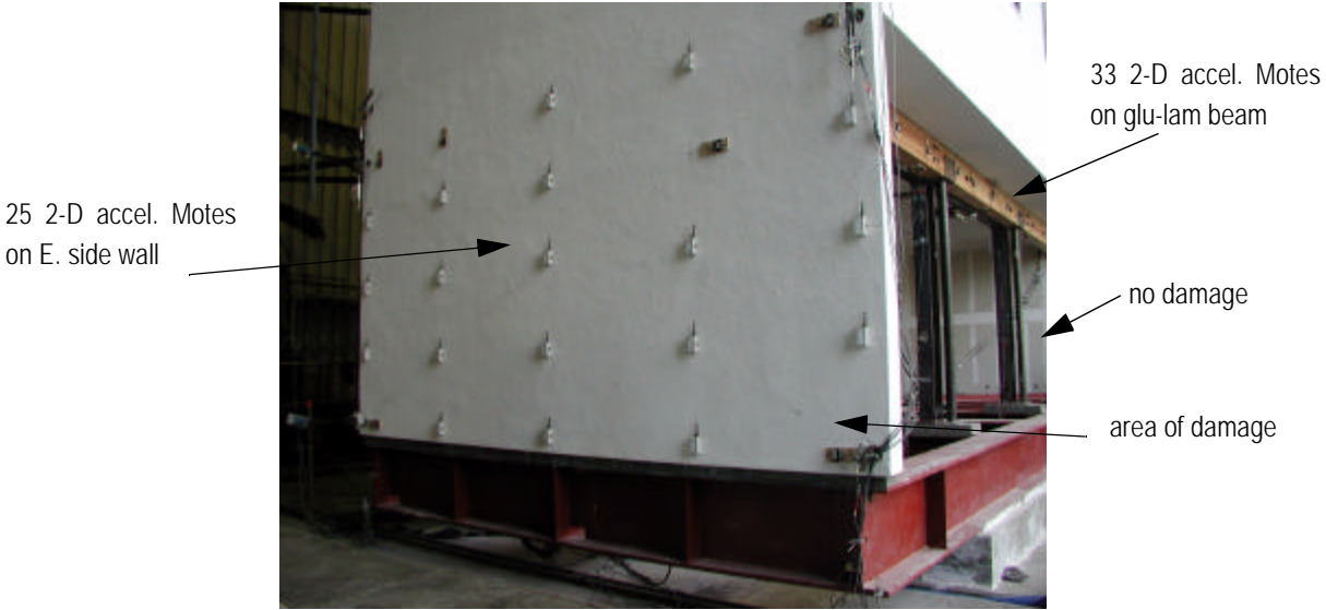
Figure 3. First dense-Pak™ instrumentation using wireless Motes on building structure. Instrumentation by Glaser on full-scale shake table test by Prof. K. Mosalam, 12/20/01.
